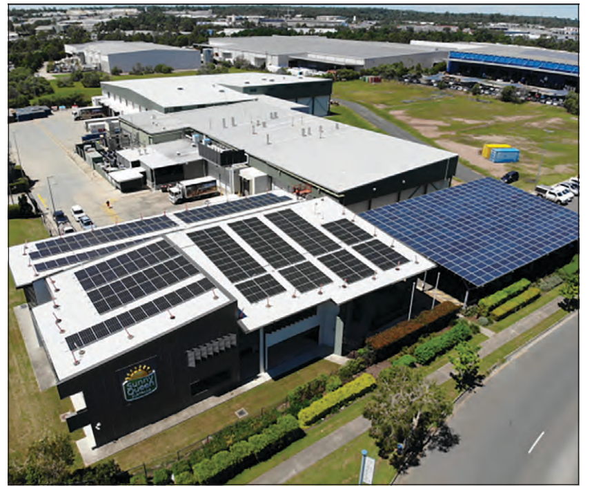
Sunny Queen has installed 626 solar panels at its Carole Park Head office to reduce carbon dioxide emissions.
