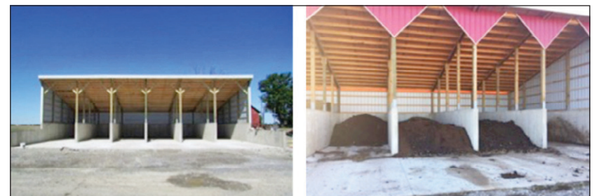
Figure 6. Examples of mortality composting bin designs Photo: blancharddemofarms.org/practices/animal-mortality-composting
